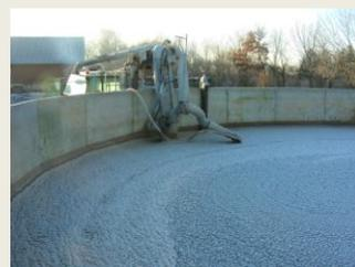
Acidification in the slurry storage is done in connection with agitating just before field application. Photo provided by HARSØ.
